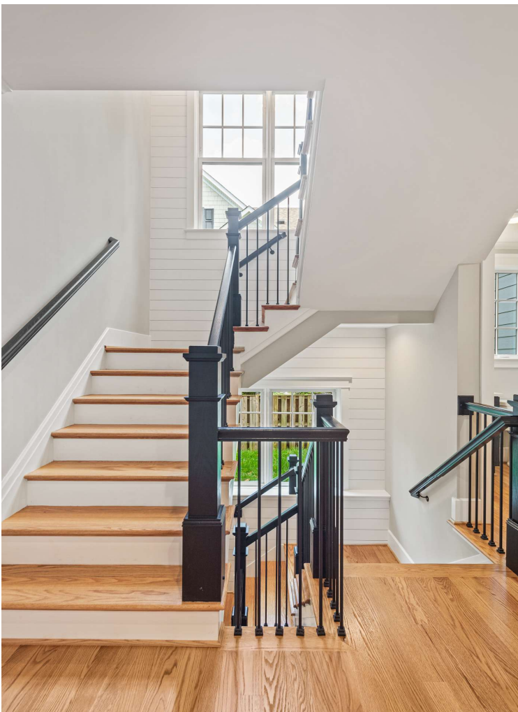
Shiplap at stairwell
